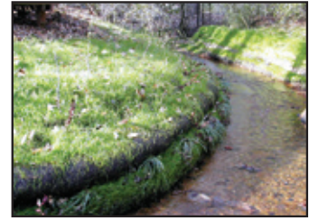
Vegetated Retaining Wall
